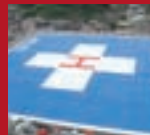
ALUMINUM HELIPORT Uwajima City Hospital
