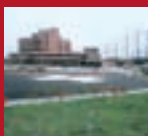
GROUND HELIPORT Awa-Ishikai Hospital
